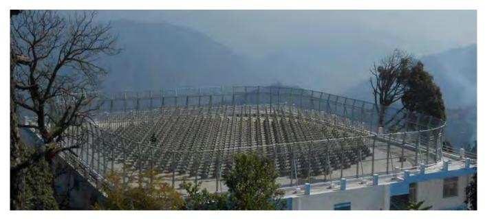
Fig. 2: Recently installed a clutter fence along the periphery of the ST Radar antenna array on the rooftop of the building.
