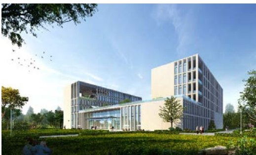
Fig. 2 Building of the Integration Information and Operation Control Center
