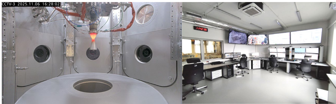
Figure 4.1.2.4. High-altitude hot-firing facility dedicated to green thruster and engine development
