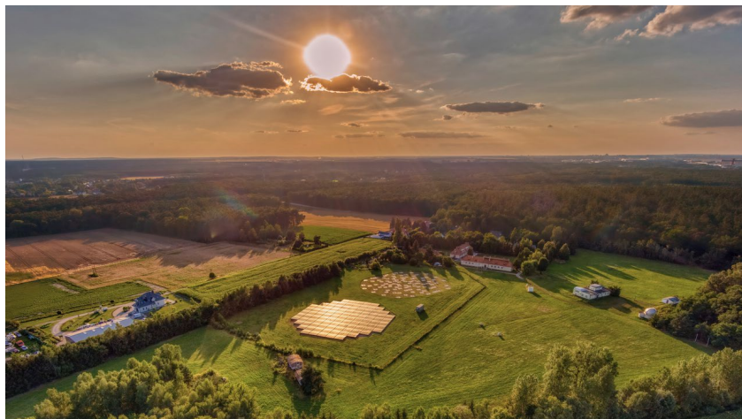
Figure 3.1.1. LOFAR PL610 station in Borówiec – aerial view
